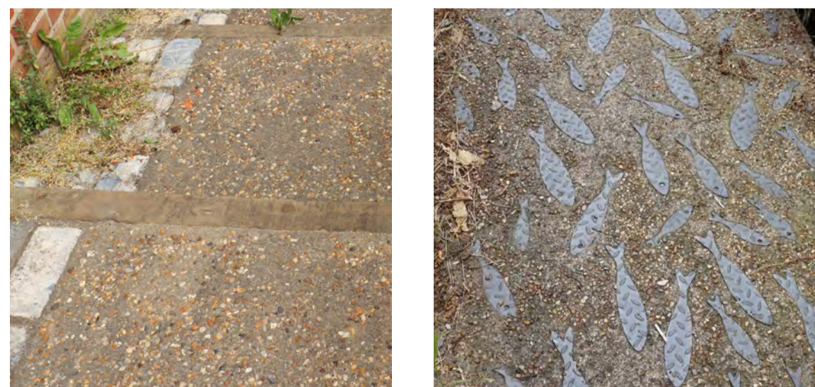
Existing In-Situ Exposed Aggregate Concrete to be repaired and cleaned
